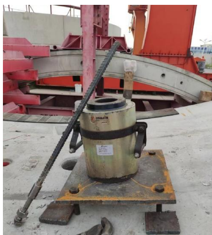
(c) 转换杆和锚杆式拉拔仪
